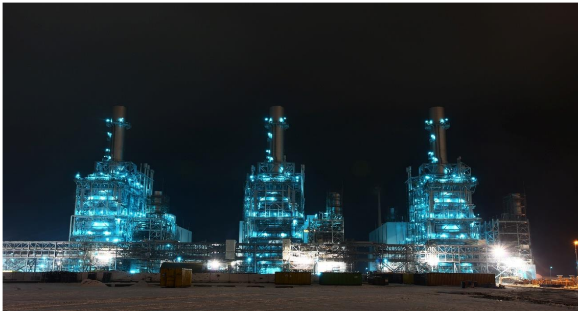
Figure 3.B: Vattenfall's gas power plant Magnum (Image by Nuon)
